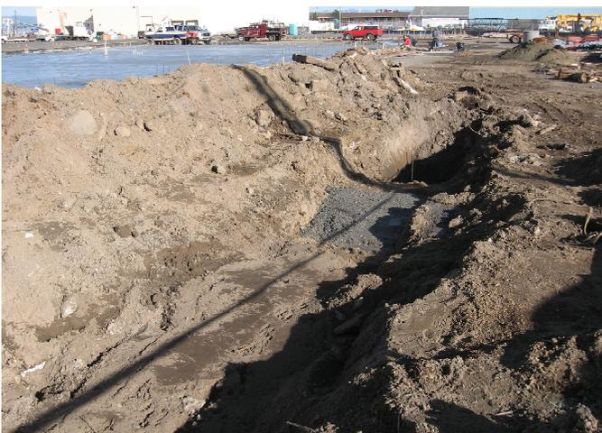
**Photo 5 - View looking NE along new sanitary sewerline trench; cofferdam in central portion of photo.**
