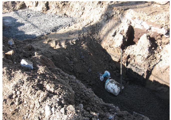
**Photo 4 - Controlled-density fill (CDF cement) cofferdam installed over and around new sewerline and gravelly fill.**
